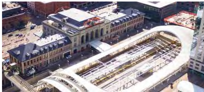
Credit: Regional Transportation District, RTD Denver
