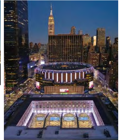
Moynihan Train Hall – Penn Station
